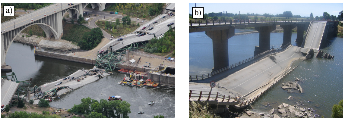
Figure 1.1: (a) Collapse of the I-35W Mississippi River bridge in Minnesota, USA, in 2007, (b) Collapse of the Loncomilla bridge in Chile in 2004.
